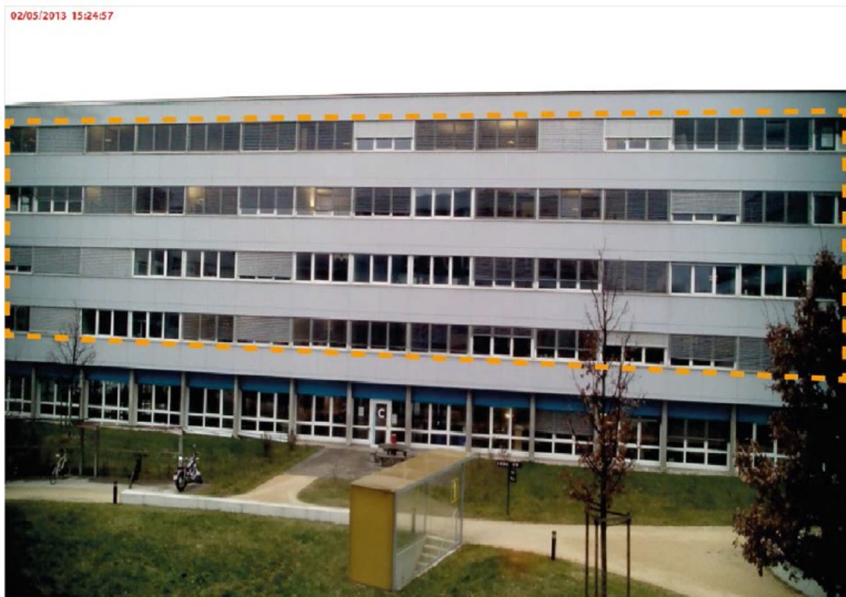
Figure 1: Photo of the west façade of building PSE-C on February 5, 2013, overcast sky
