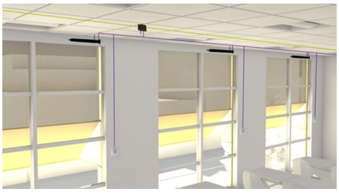
**USB** io Transceiver to integrate motors and local controls
